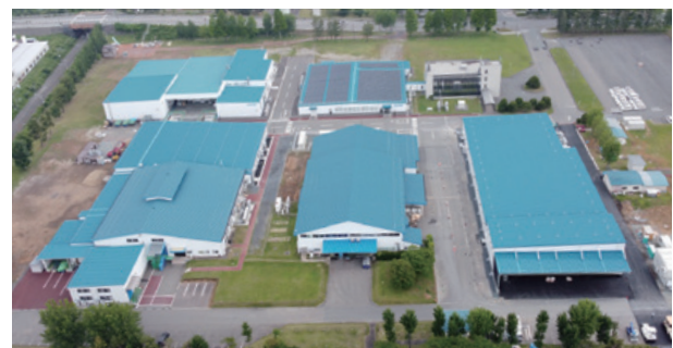
Our production facility under expansion (Kitakami, Japan)
